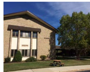
Contini Hall (pictured) received mechanical, lighting and IT upgrades in summer 2015.
