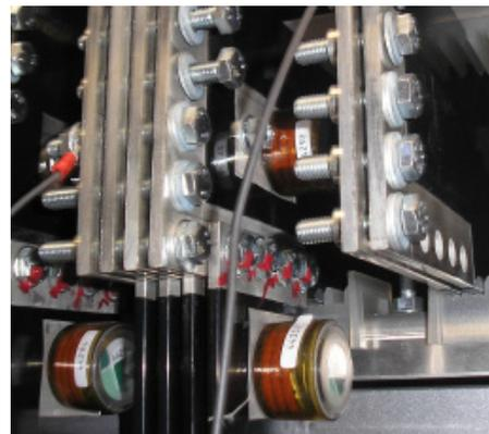
Photo shows the placement of temperature monitor sensors attached to service entrance bussing.
