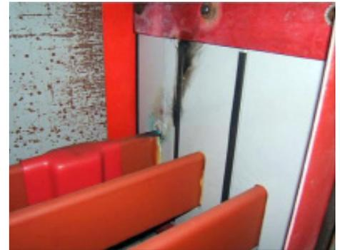
Photo shows clear indications of corona tracking due to damaged insulation laminate on bussing and long term electron tracking prior to a phase-to-ground fault condition.
